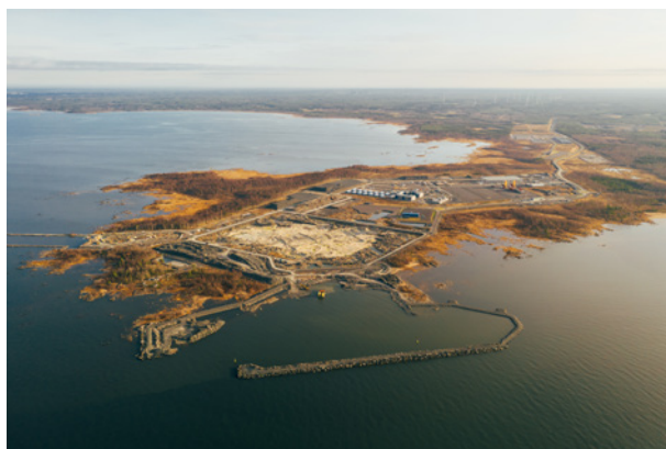
Hanhikivi 1 site in Northern Finland © Fennovoima
