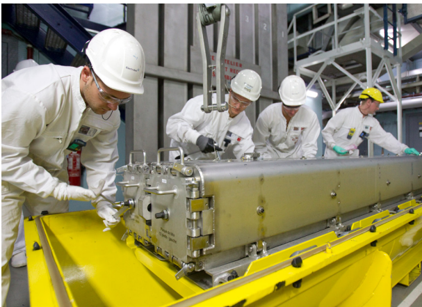
Fuel assembly handling Tihange NPP ©Synatom
